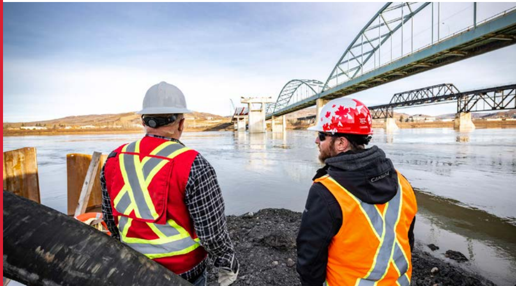
📍 Peace River Bridge Twinning
