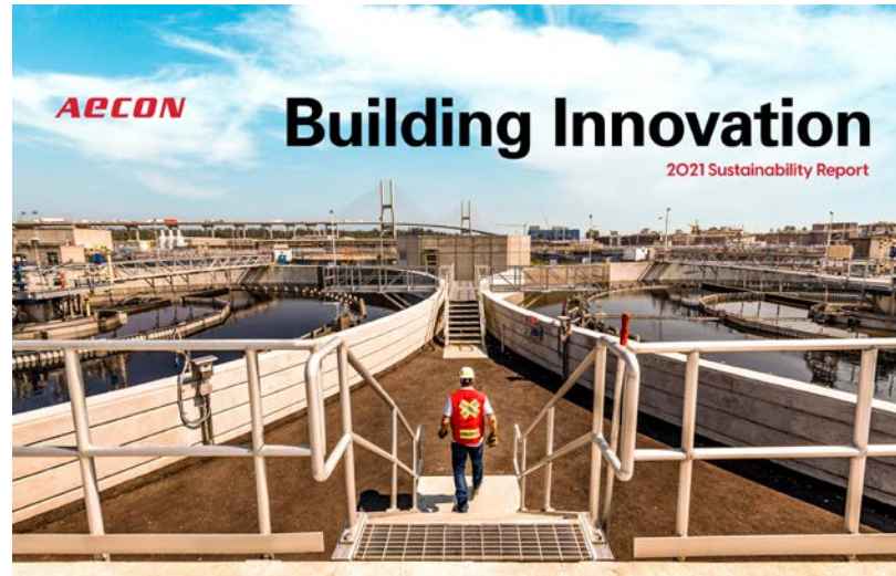
Annacis Island Wastewater Treatment Plant
