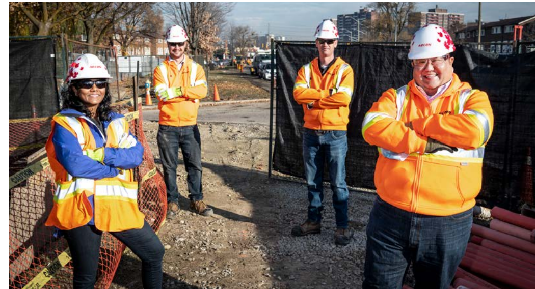
📷 Aecon employees at a Telecommunications project site
