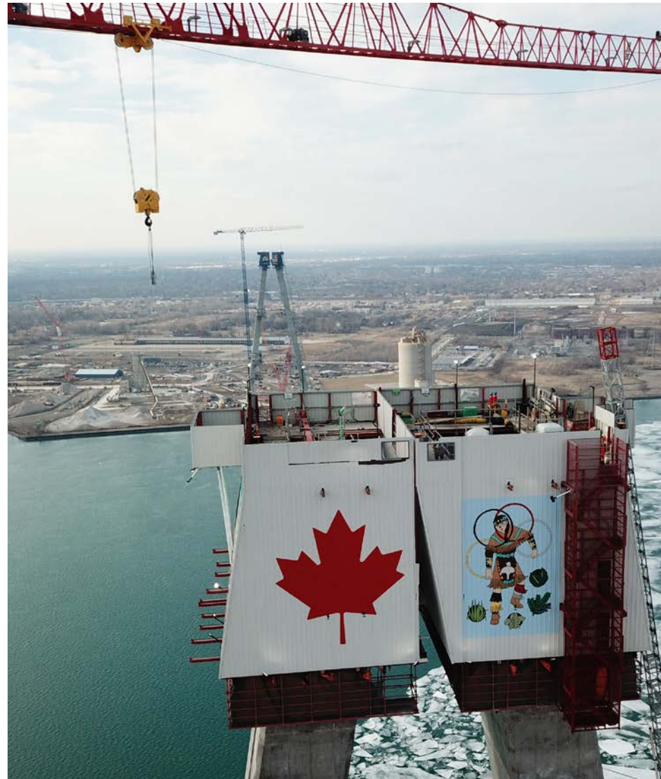
📷 Ongoing construction of the Gordie Howe International Bridge
