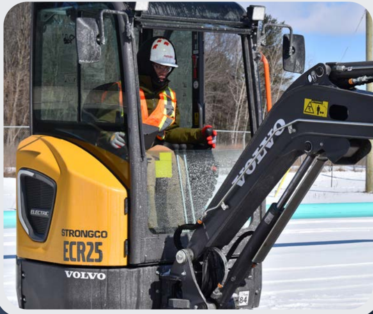
📍 Aecon employee using an electric mini excavator, Ontario
